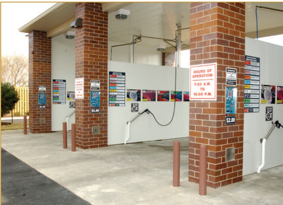
Clean bay walls as well as instructional boards aid in the overall appearance of your site.
